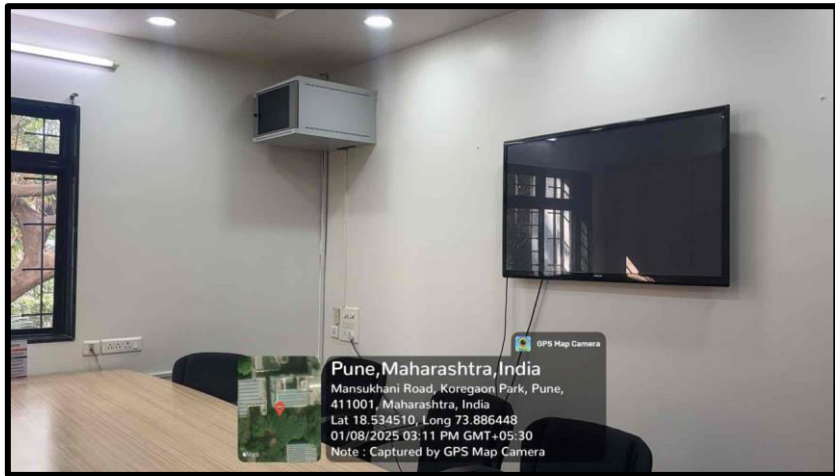
Yamaha Mixer with JBL Speaker, M Track Audio Interface Installed at Patio
